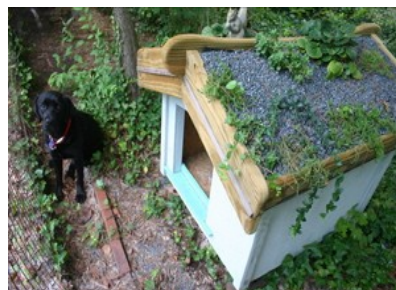
Picture shows a newly planted roof. As plants mature the open spaces will fill in.
